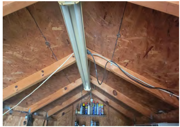
66 Tool Shed Roof Framing
