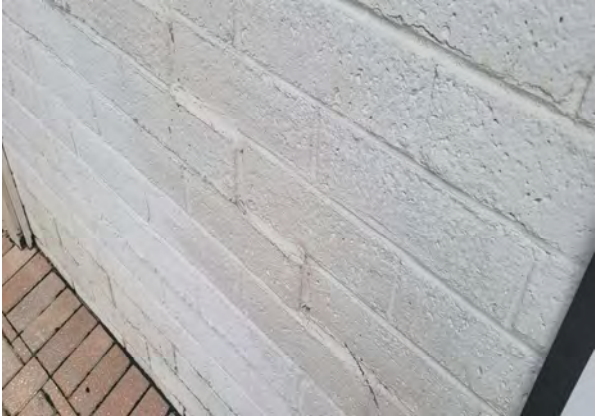
51 Exterior Side of Bicycle Storage Room Wall
