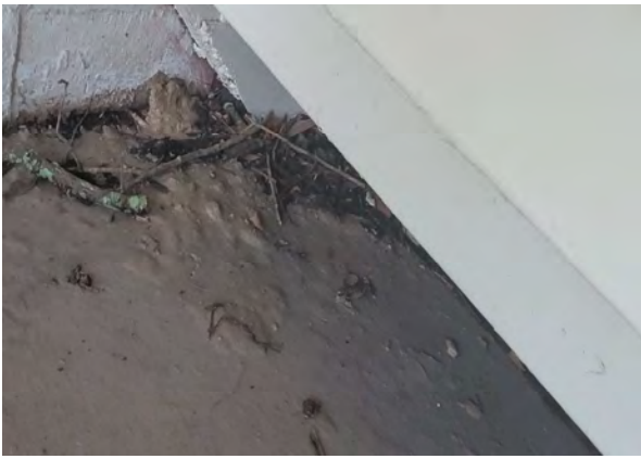
73 Hallway F Rust at Stairs
