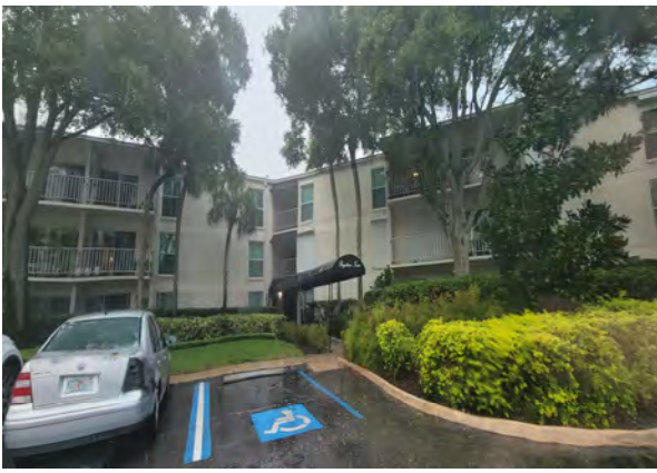
1 Front of Building
