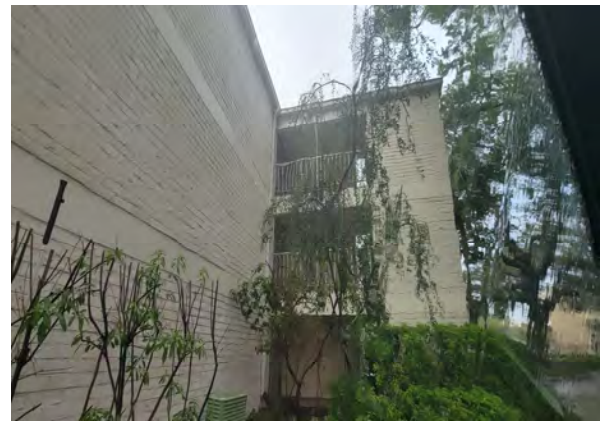
2 Right Side of Building
