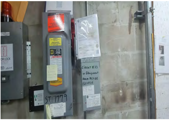
33 Elevator Disconnect
