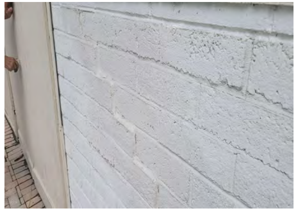
50 Exterior Side of Bicycle Storage Room Wall
