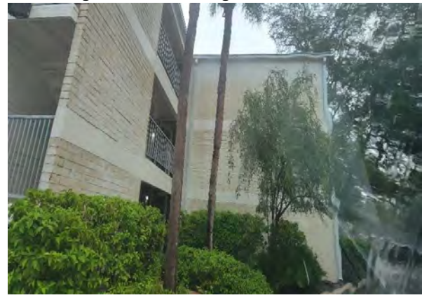
4 Left Side of Building
