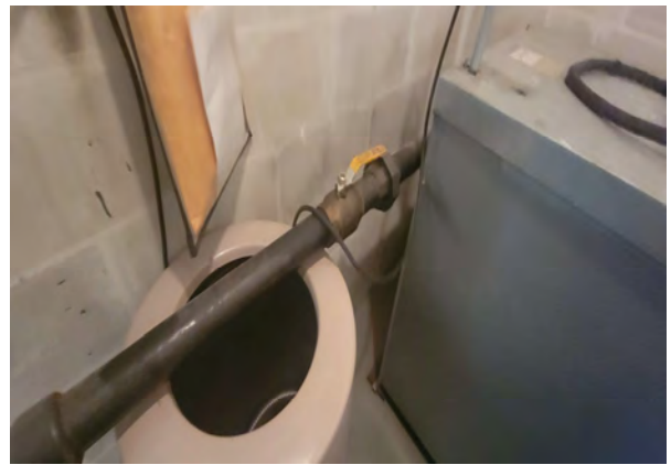
22 Elevator Motor Disconnect
