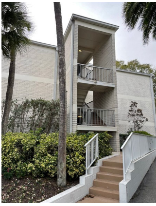
1 Stairwell A overview
