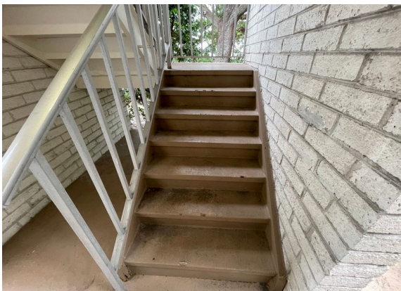
23 stairwell B steps
