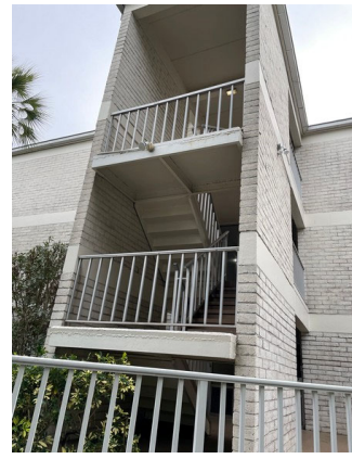
2 Stairwell A overview
