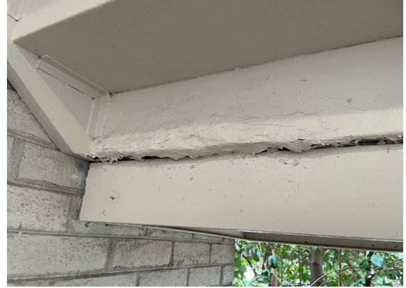
20 stairwell B corrosion
