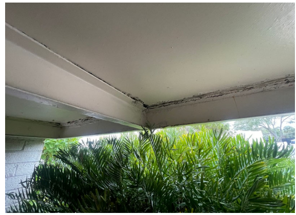
34 stairwell F corrosion
