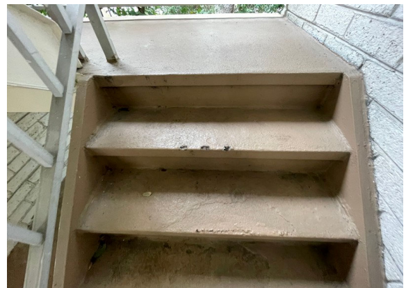
24 stairwell B steps
