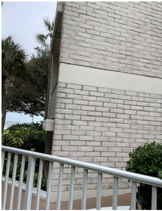
3 Stairwell A overview
