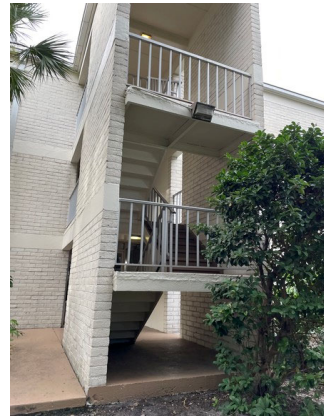
14 stairwell B overview
