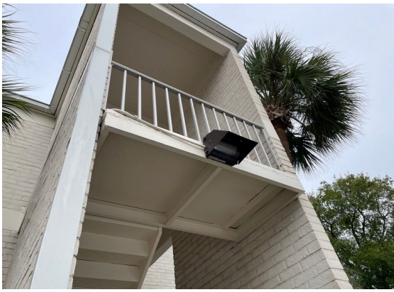
33 stairwell F overview
