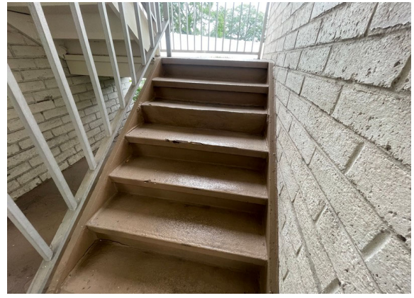
42 stairwell F steps
