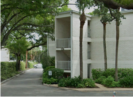
27 stairwell E overview
