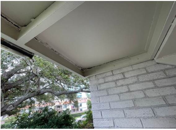
25 Stairwell B 2nd level landing overview
