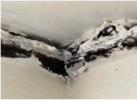
9 stairwell A corrosion
