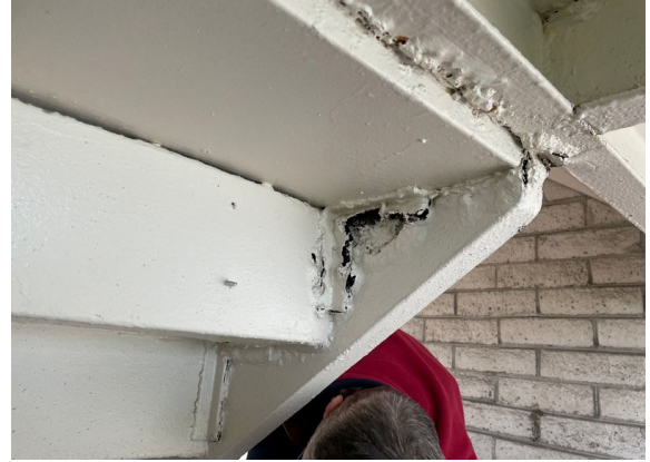
10 stairwell A corrosion
