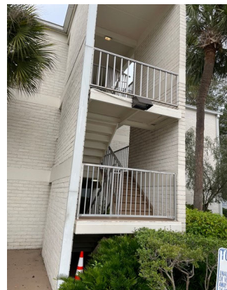
32 stairwell F overview
